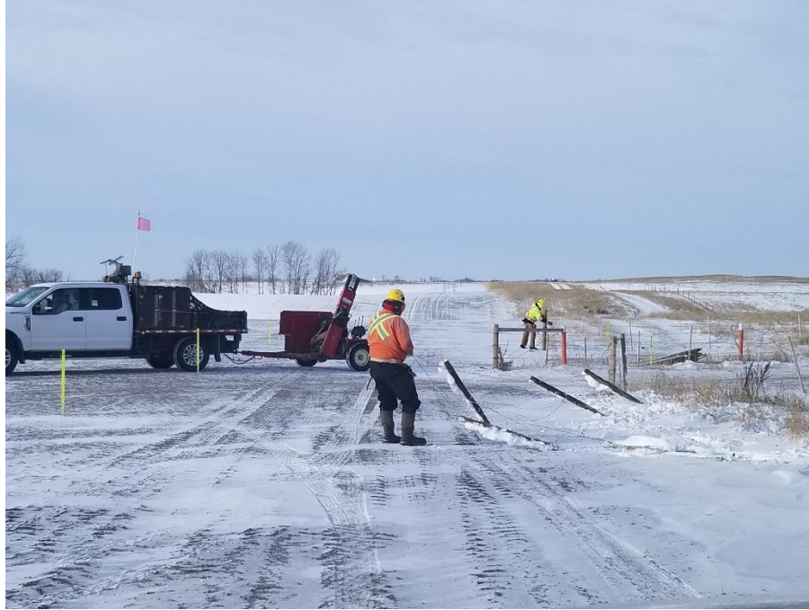
Utility crew installing fence pounding posts into frozen ground.
