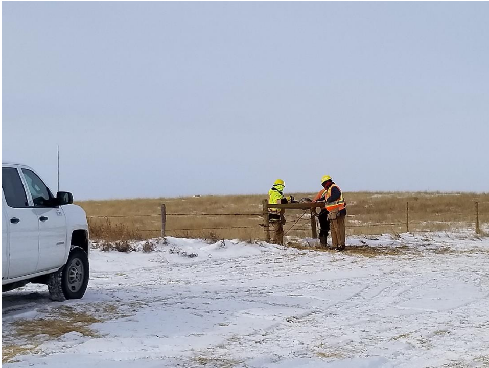
Utility crew fixing and adding a brace for the fence.
